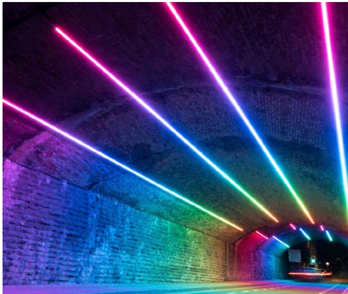
Hood Road tunnel light installation (Flow) designed by Jessica Lloyd-Jones in collaboration with Architainment
